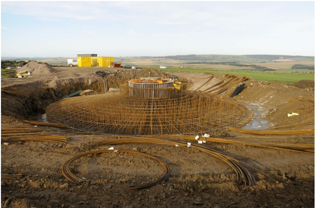
Image below: early construction phase of an industrial turbine base
